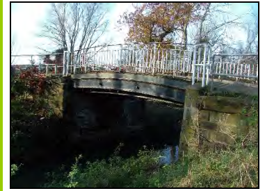
The Navigation Bridge
