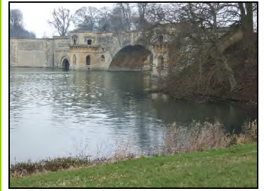
The Blenheim Bridge
