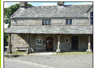
Church House Widecombe
