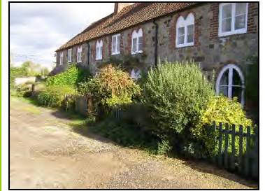
Mill Workers Cottages
